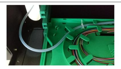
9. Splice the fiber cable with pigtails in the tray. Insert the heat shrinkable protective tube into the slots in the middle of splice tray. Coil the redundant fibers in the splice tray.
