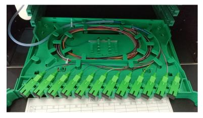
10. After finishing splicing fibers and coiling the redundant fibers, make record on the fiber port diagram inside the front door and then push back the tray into ODF. Close the front door of ODF when all jobs are finished.
