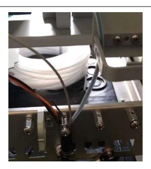
6. Insert fibers together with protection loose tube from the inlet cable holes on the left or right sides of ODF. Use screwdriver to poke a hole on rubber gland or just remove the rubber gland to insert the fibers with protection tube.
