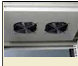
Cabinets are vented to allow cooling
